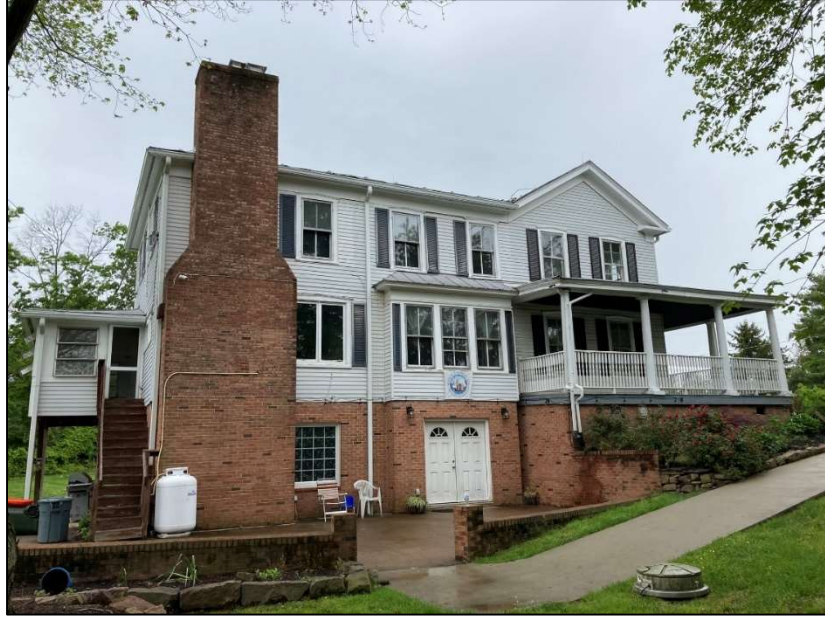
Figure 17. Sunnyside House, east elevation. May 2023. Photo by the author.
