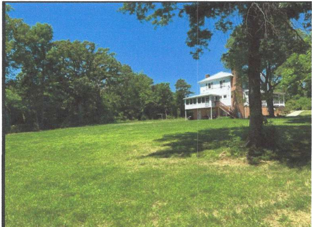
F-6: Rear Yard of Existing Building to be demolished.
