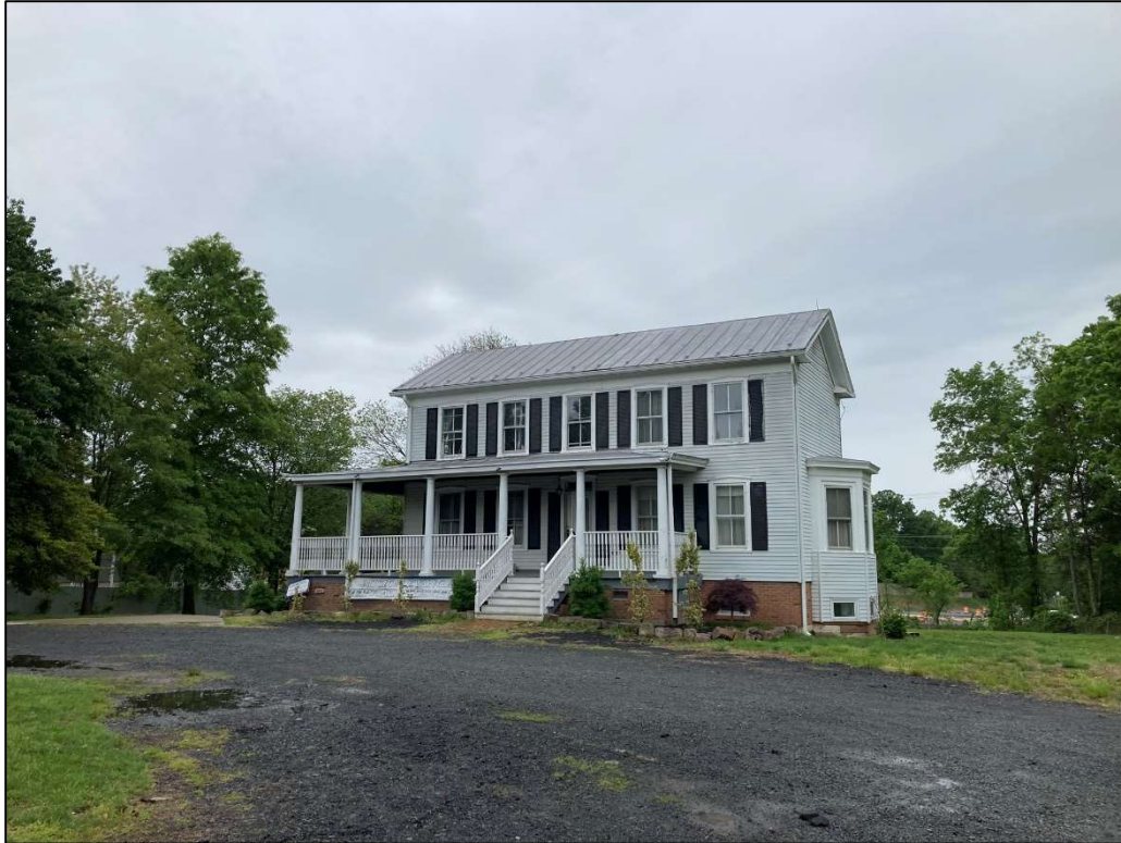
Figure 12. Sunnyside House, northwest oblique, May 2023. Photo by the author.
