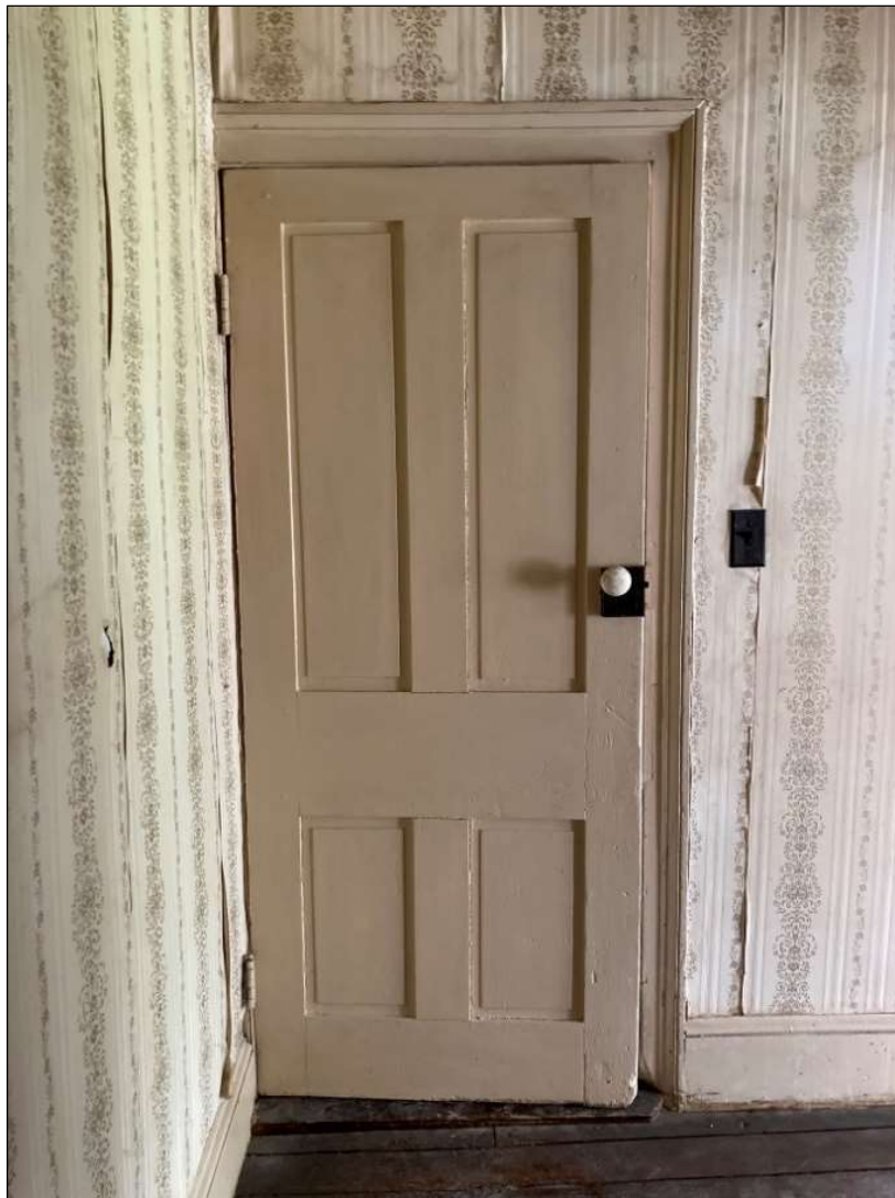
Figure 69. Door between rear hall (log section) and kitchen, view from rear hall. May 2023. Photo by the author.
