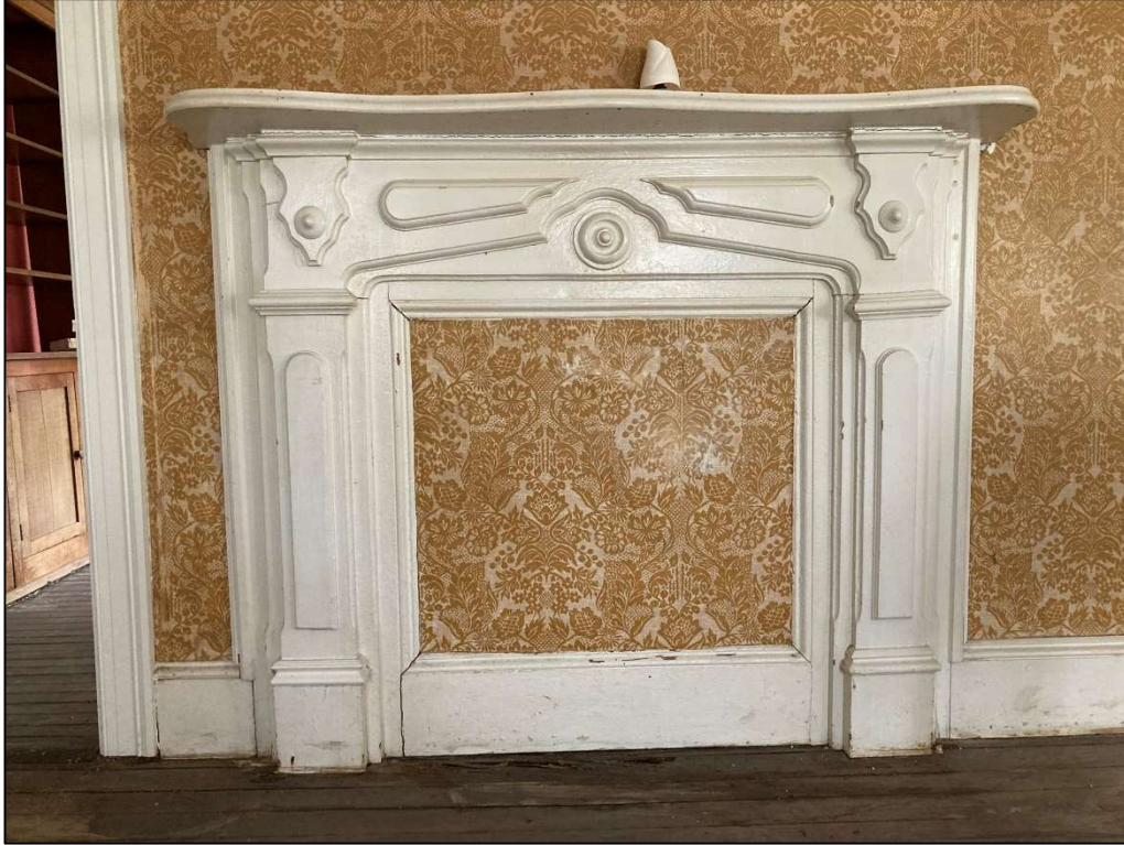
Figure 25. Mantel, west front room. May 2023. Photo by the author.
