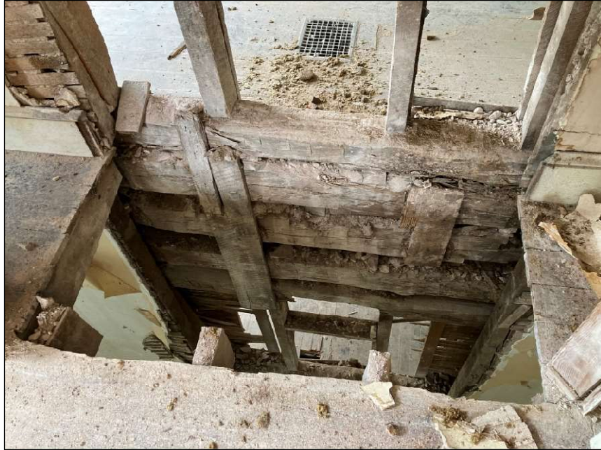
Figure 47. Second floor, looking down where the stone chimney used to be. May 2023. Photo by the author.
