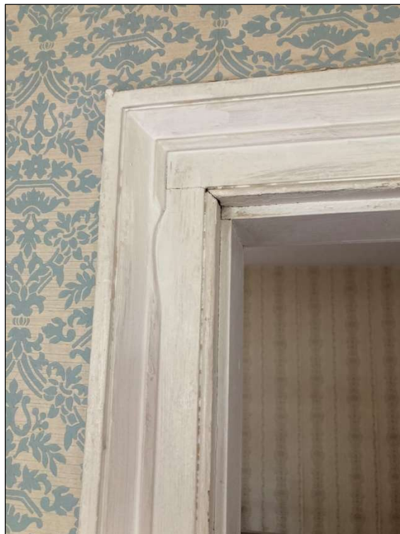
Figure 71. Second floor, door trim around the inside of the doorway between the rear hall and the bedroom (log section). May 2023. Photo by the author.
